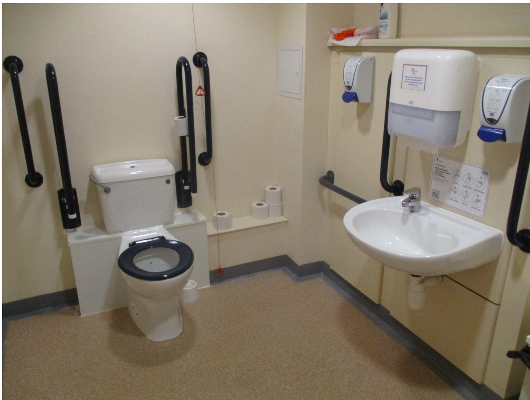
Photo 25 Peninsular layout accessible WC facility.
