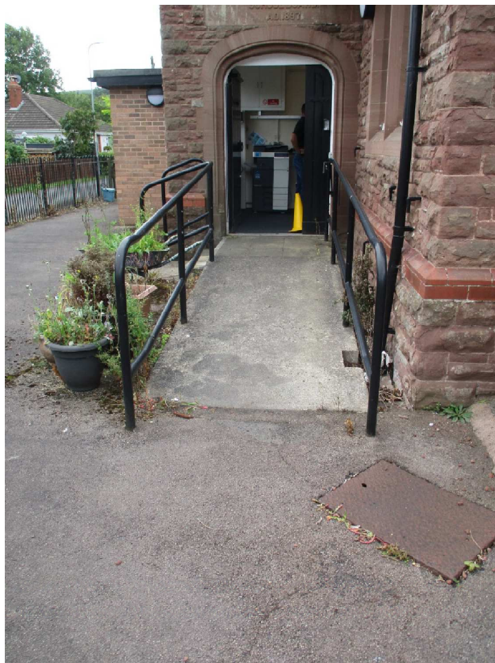
Photo 15 – Entrance ramp/ steps
