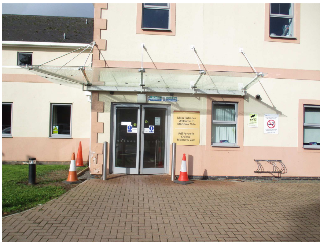
Photo 27 Level entrance/ automatic entrance doors.
